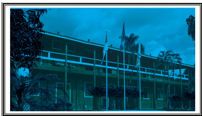
Fachada principal – Museu Palacinho
